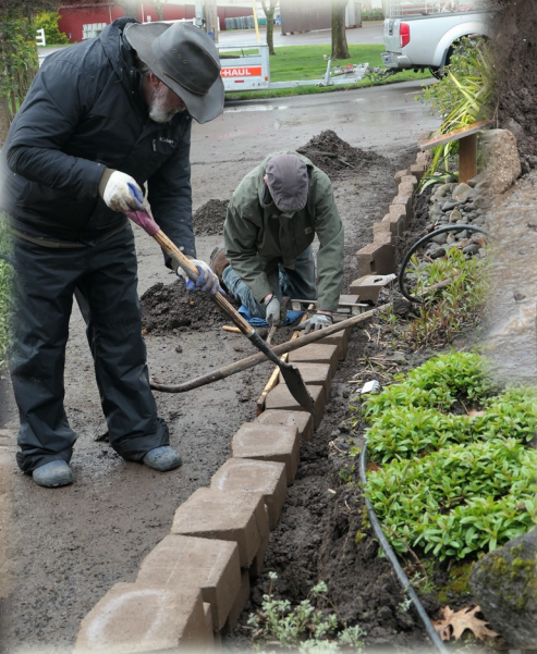
Dennis laid the foundation layer for the whole wall. 3 hours on his knees...
