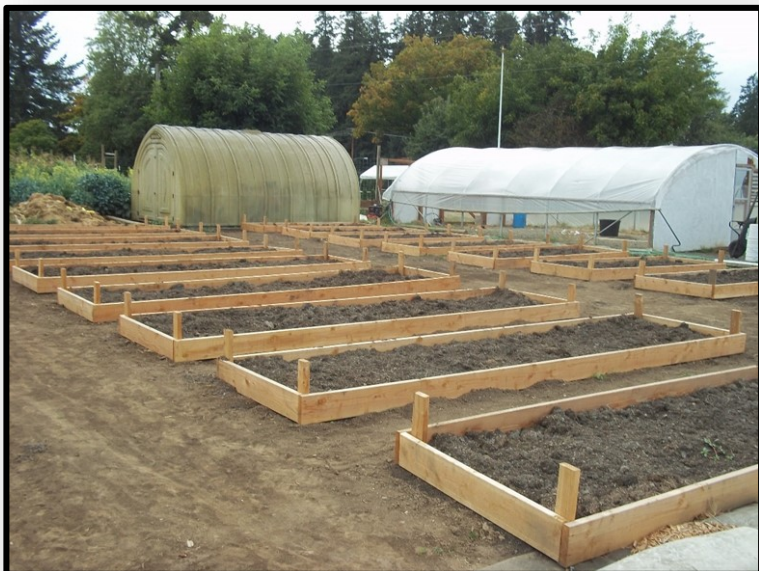
Newly-constructed beds and the greenhouse.
